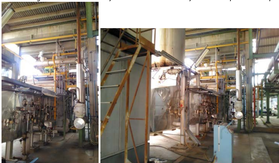
Figure 1 - Exhaust gases vent and recovery boiler - Co-Generation System - Campoverde di Aprilia Plant
