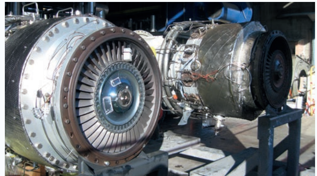
Figure 2 Installation of the gas turbine into the system, August 2016
