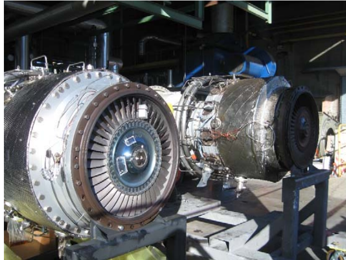
Figure 2 - Installation of the gas turbine into the system, August 2016
